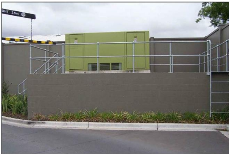
Figure 51 - Example substation raised above 1:100 flood level
